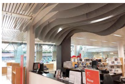
Acoustic treatment, State Library of NSW
