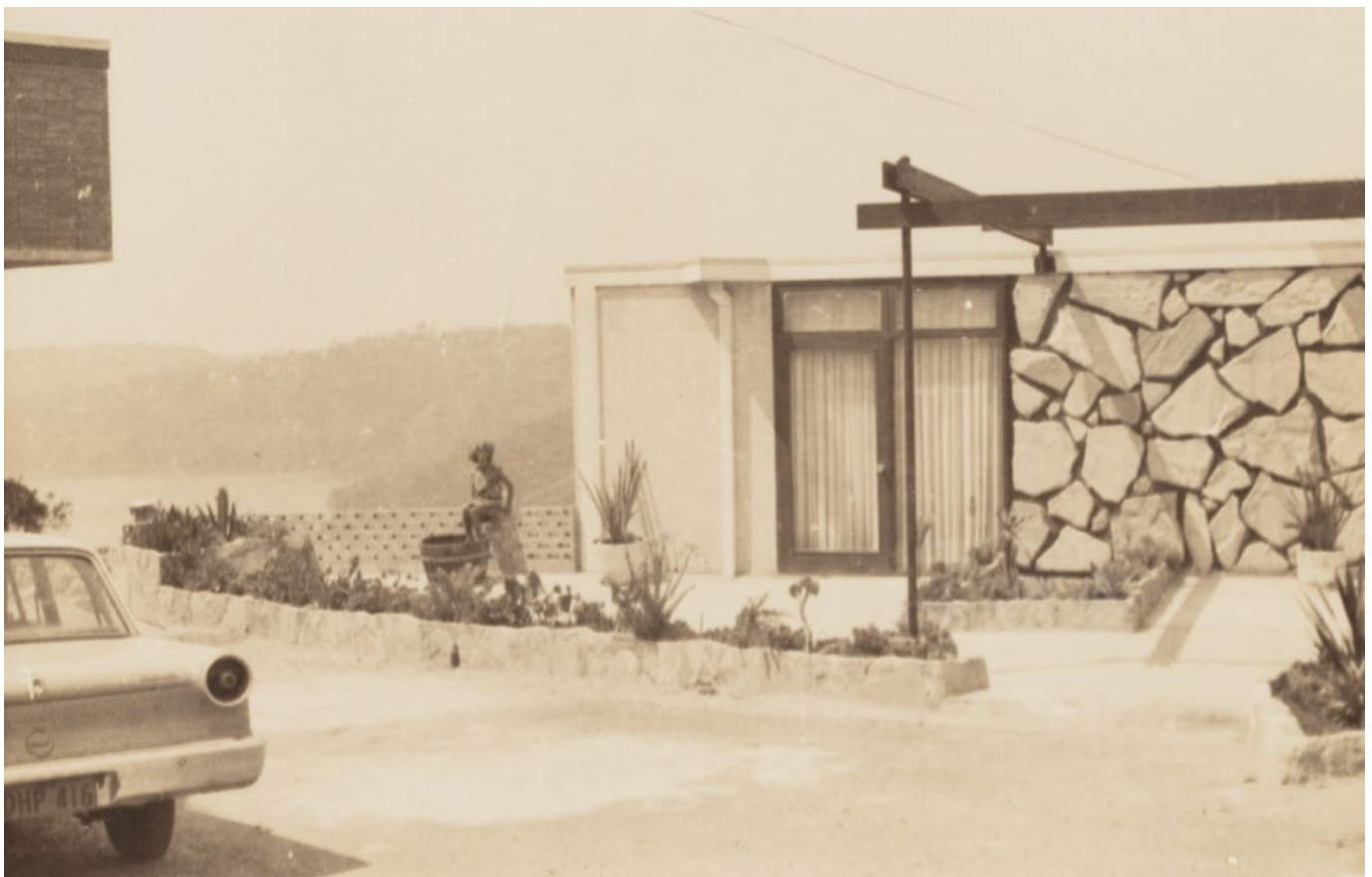
Design for the 'Beachcomber' project home, Nino Sydney for Lend Lease Homes, c 1961 Exterior, Nino Sydney designed project home, 1960s
