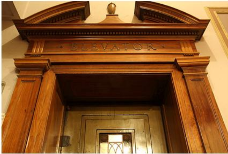
The lift was installed in 1930 – photo by Peter Ittak, 2014
