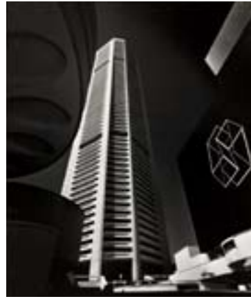
ABOVE: MLC CENTRE, SYDNEY, HARRY SEIDLER & ASSOCIATES, 1972-1975, MAX DUPAIN (PERMISSION OF PENELOPE SEIDLER AM), PXB 237/61
